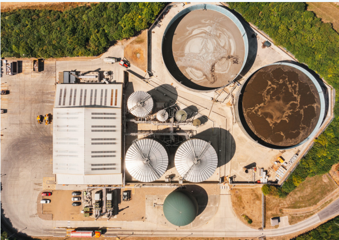
Recycling center for biomass – example for the use of the proceeds of a Green Loan
